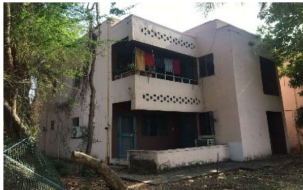
Figure-10: Stagnant PNG pipeline at nearby by building
